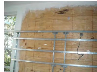
EXAMPLE - PLYWOOD SHEATHING
