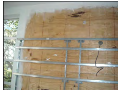
EXAMPLE - PLYWOOD SHEATHING
