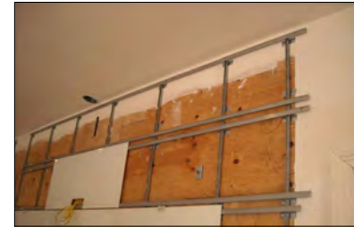
EXAMPLE - PLYWOOD SHEATHING
