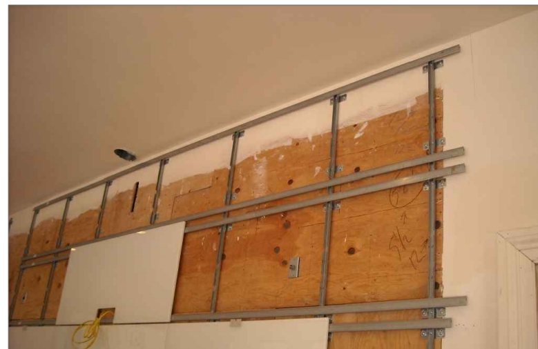
EXAMPLE - PLYWOOD SHEATHING
